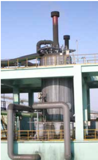
Fig. 3: Degassers at a COREX® plant for forced degassing of process water return
