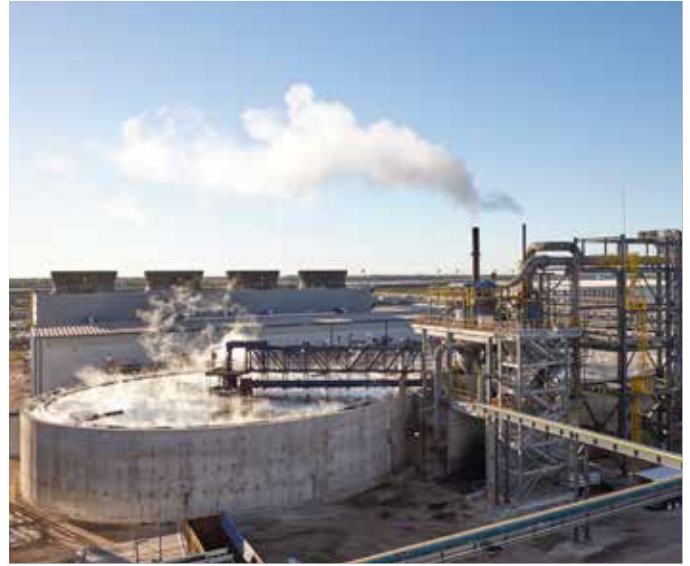
Fig. 2: Degassers for Midrex top gas scrubber weir return and top gas scrubber cone return (to the right of the clarifier)
