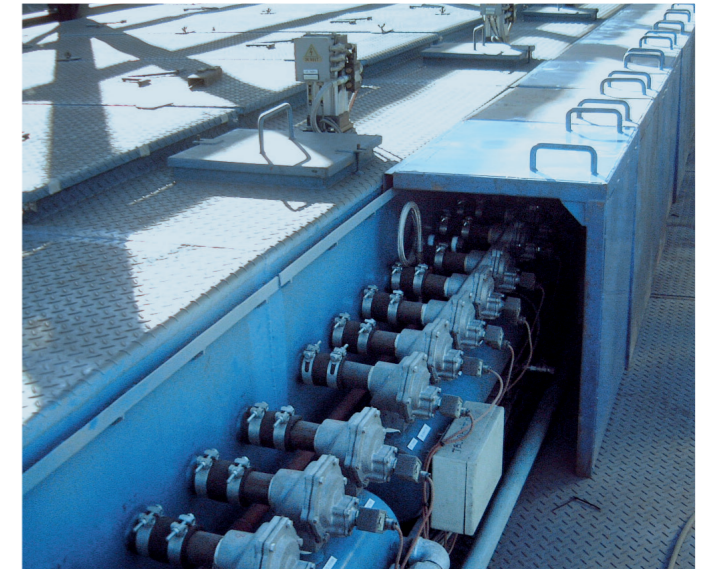
Pulse jet valve arrangement with noise cover
