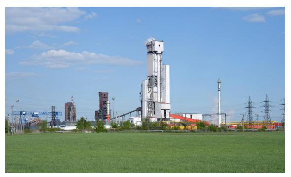
Midrex direct reduction HBI plants of Lebedinskiy GOK near the city of Gubkin, Belgorod Region, Russia (Midrex HBI-3 in the front, Midrex HBI-2 in the middle and HYL HBI-1 in the background). The largest single module of this type in Russia was built by Primetals Technologies and Midrex Technologies, Inc. and achieved the performance test certificate on June 30, 2017.
