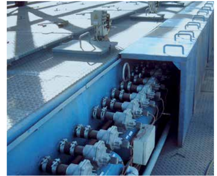
Pulse jet valve arrangement with noise cover
