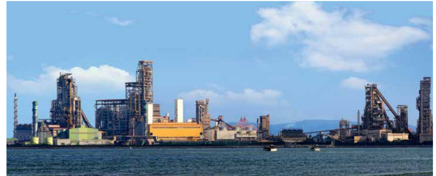
The FINEX® F-1.5M plant and FINEX® Demonstration Plant at POSCO Pohang
