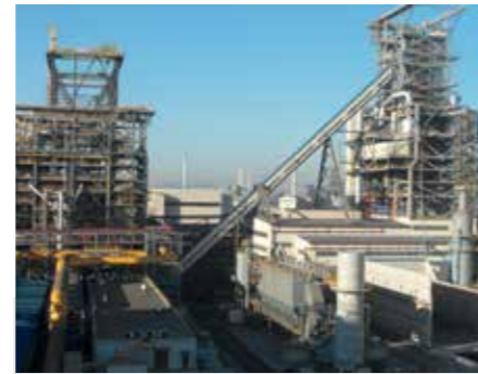
POSCO POHANG WORKS (KOREA) - FINEX® F-2.0M PLANT
