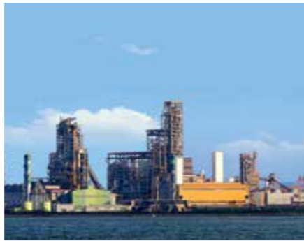
POSCO POHANG WORKS (KOREA) - FINEX® F-1.5M PLANT
