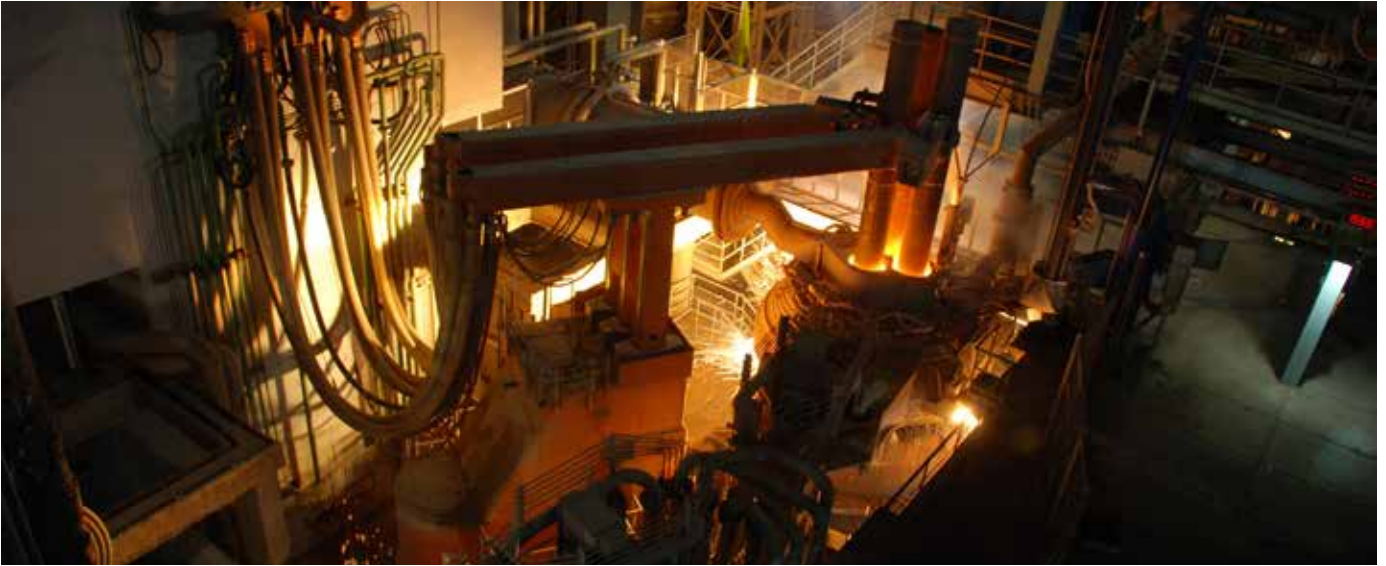
180t Twin LF, Taiyuan Iron & Steel. Co. TISCO, Taiyuan, China
