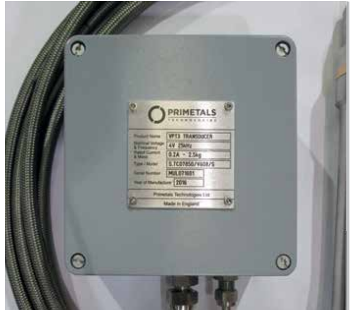
Junction box for direct wiring
