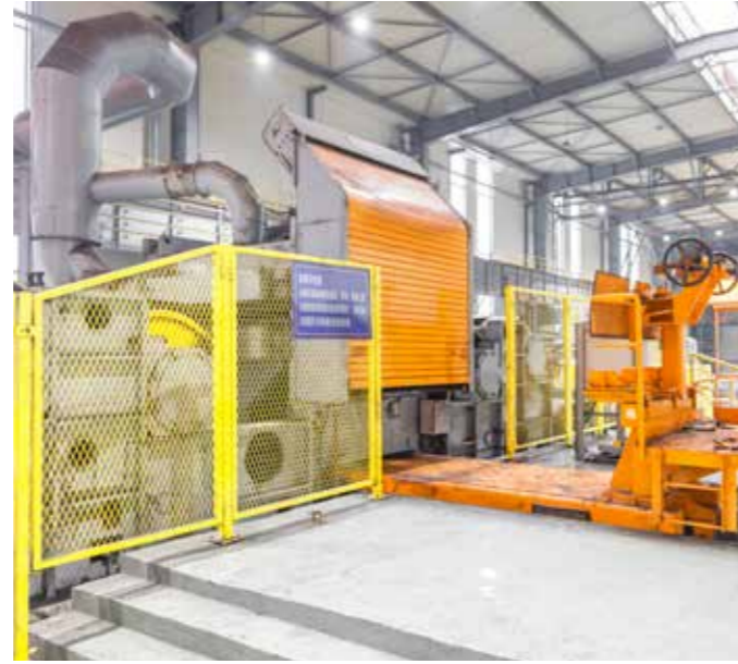
SB 75, Pickling line tandem cold mill
