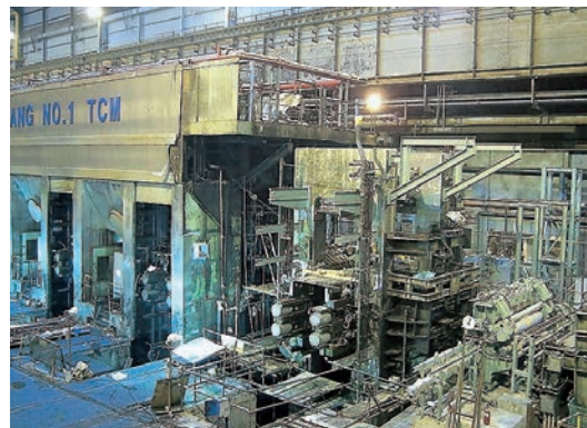
Installation of No.0 stand ( UCMW )
