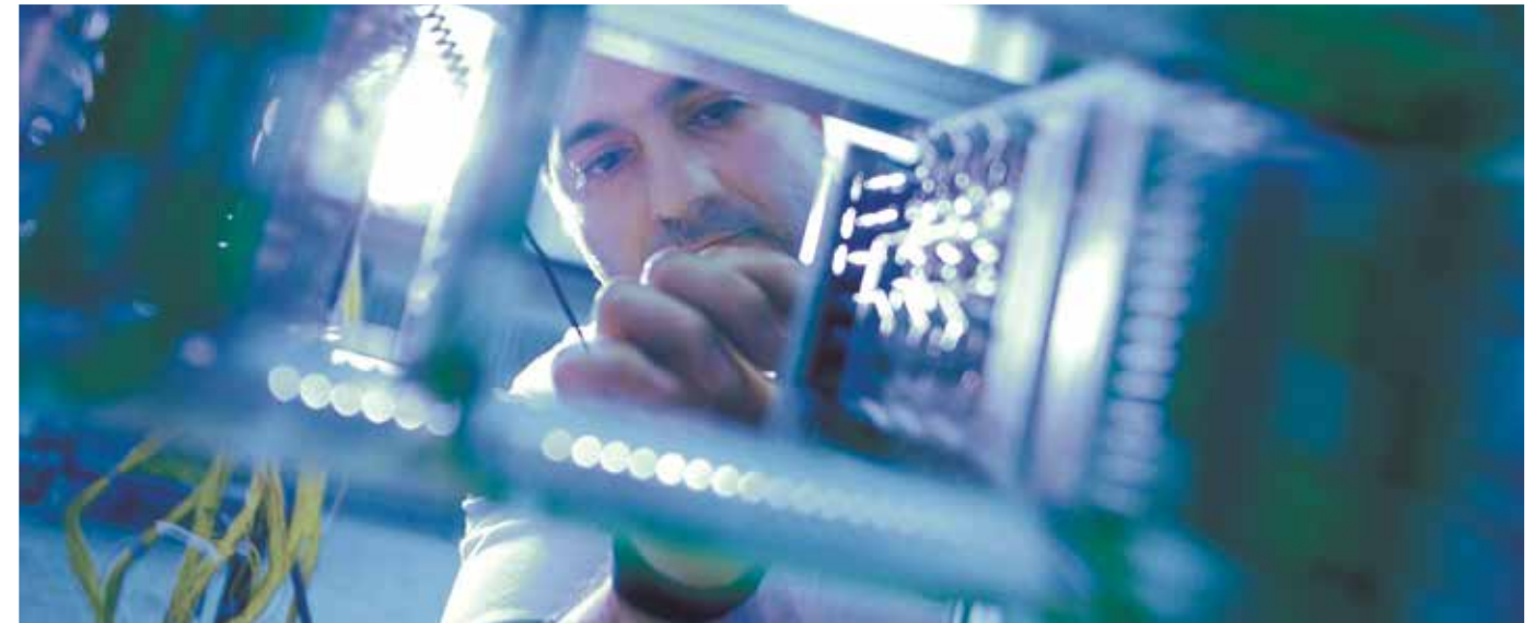
Component check in a PLC
