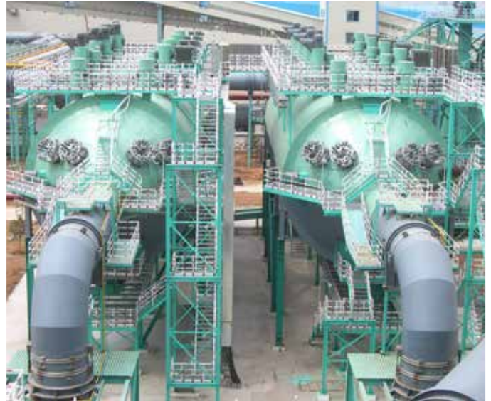
Electrostatic precipitator (ESP)
