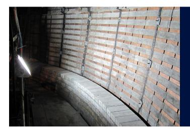
Wear-resistant solution used to overcome poor internal furnace line design.
