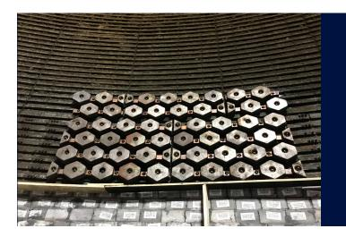
A novel solution which enabled wear-resistant inserts to be installed on existing staves.
