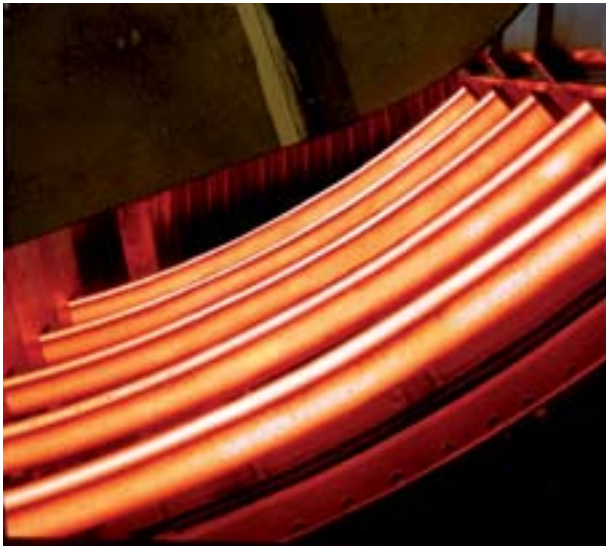
5-strand bloom caster installed by Primetals Technologies at voestalpine Stahl Donawitz GmbH, Austria
