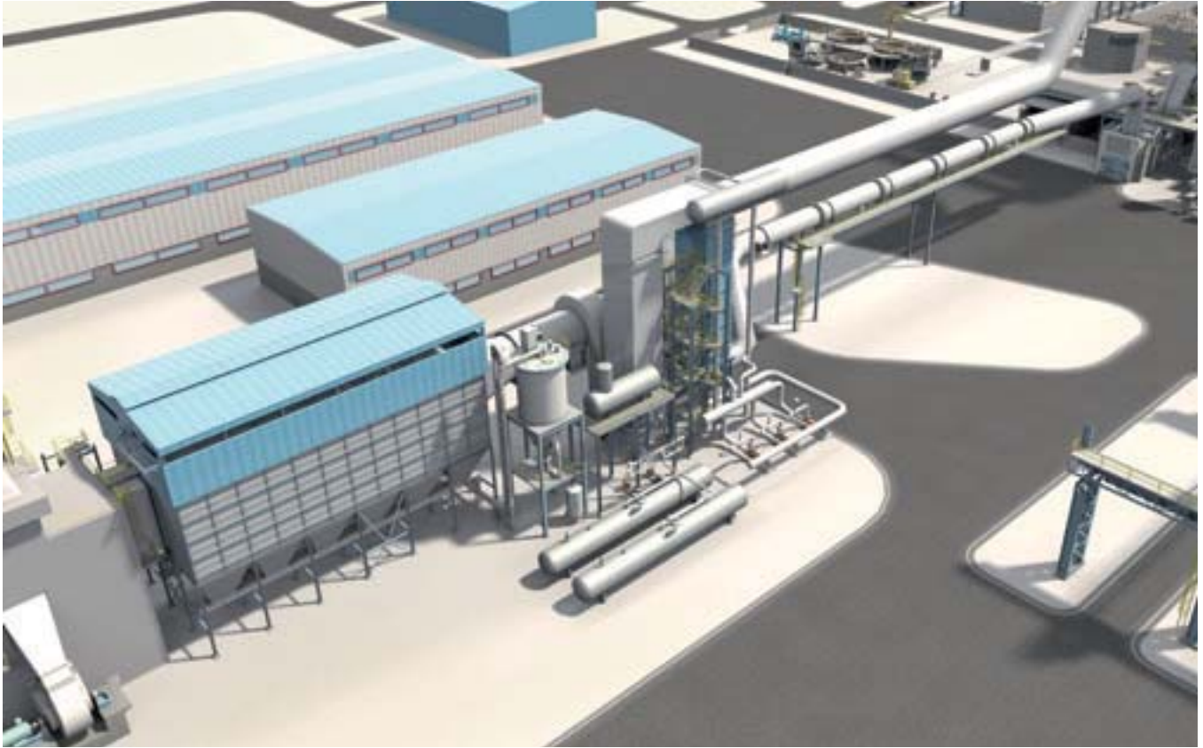
Schematic view of a waste-heat recovery system for an electric arc furnace
