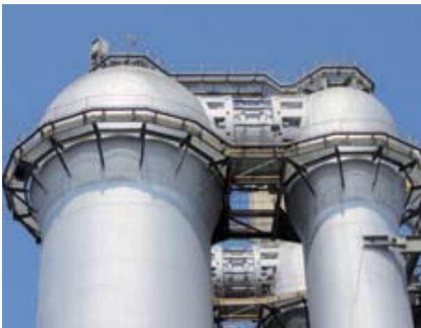
External stove crossover of the hot-blast system from Primetals Technologies
