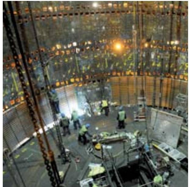
Cooling-stave arrangement in the blast furnace
