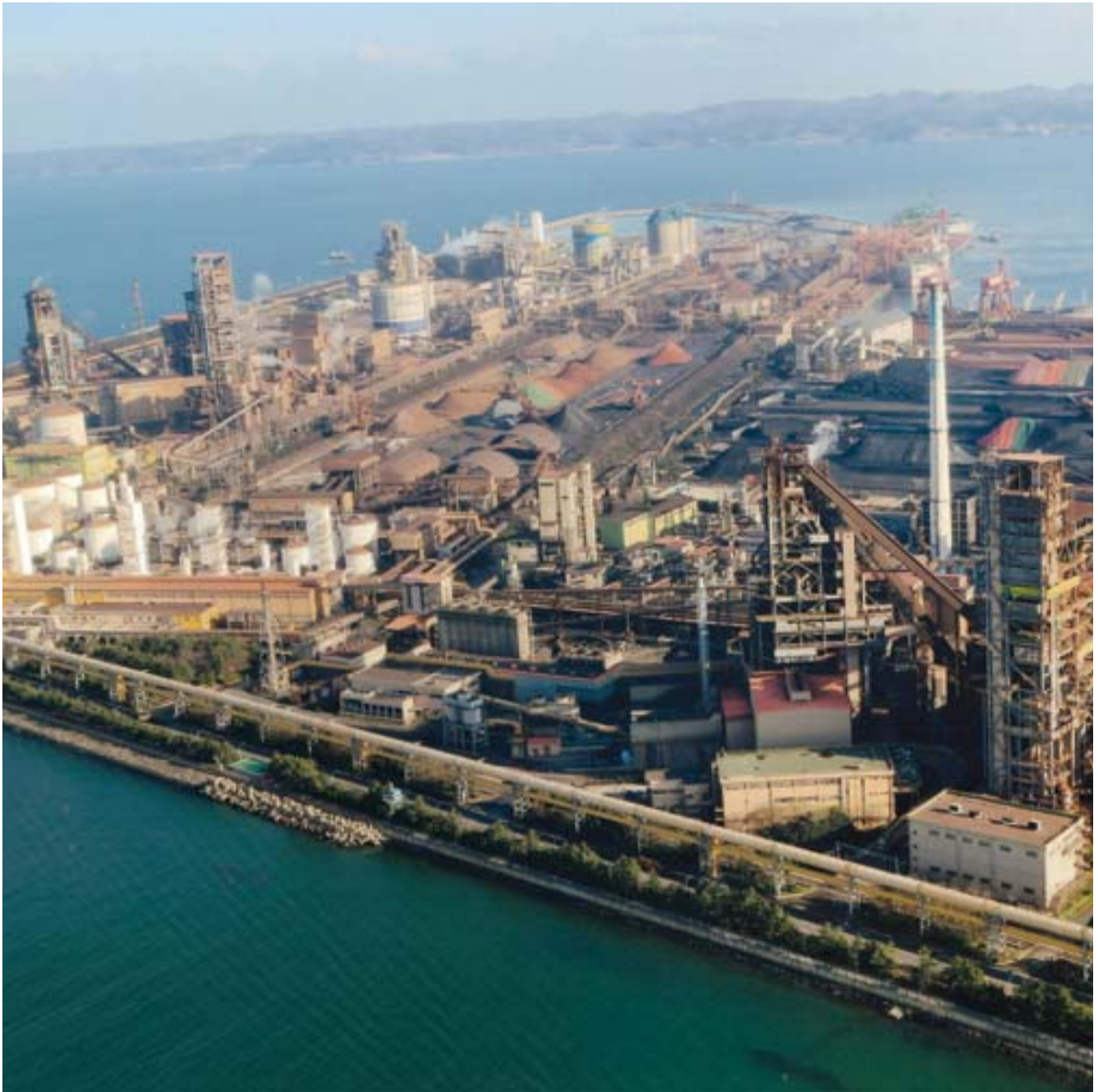
Aerial view of Posco's Pohang steelworks with three Finex plants; right: Finex F-2000 Demonstration Plant (approx. 800,000 t/a), left: Finex 1.5M (1.5 million t/a), center background: Finex 2.0M Plant (2 million t/a)
