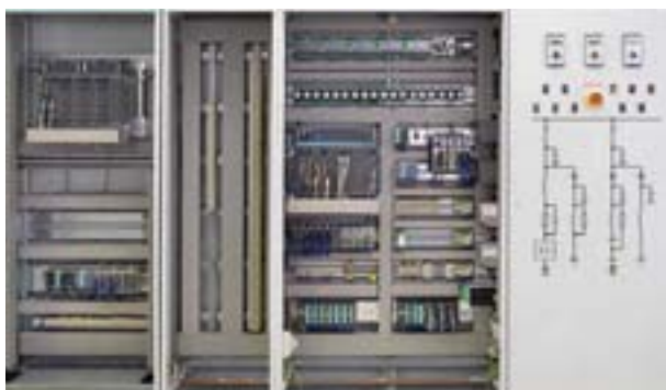
SVC PLUS control cubicle based on Simatic TDC
