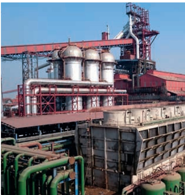
View of the new Blast Furnace No. 1 at the Kalinganagar steelworks of Tata Steel Ltd. - the largest blast furnace in India
