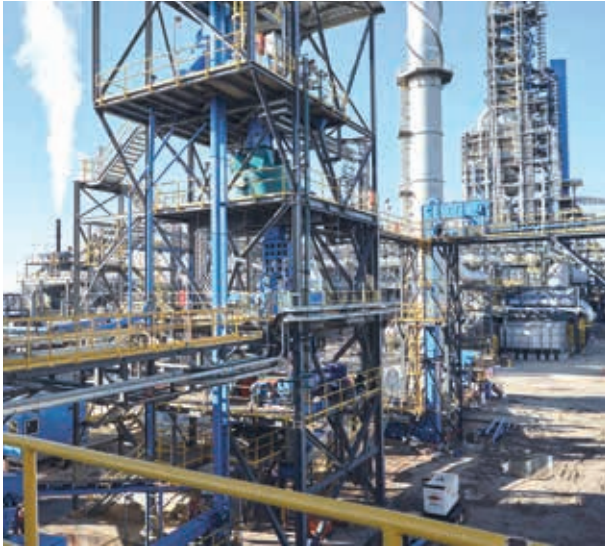
Example of a ferrous by-production recycling plant supplied by Primetals Technologies
