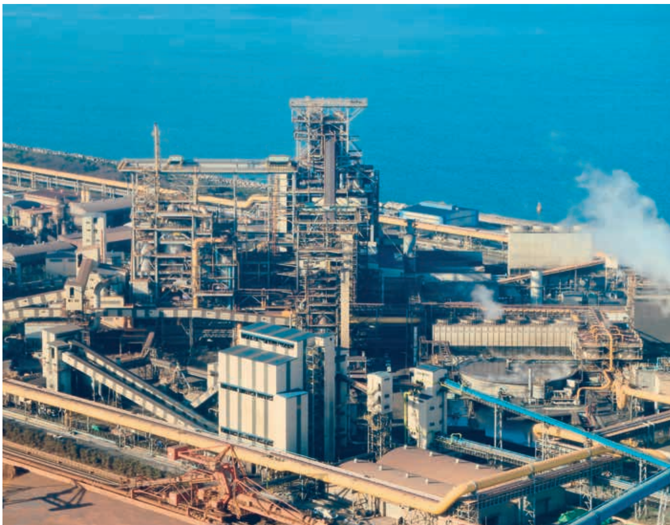
Aerial view of the Finex 2.0M plant with a nominal capacity of 2 million ton of hot metal per year
