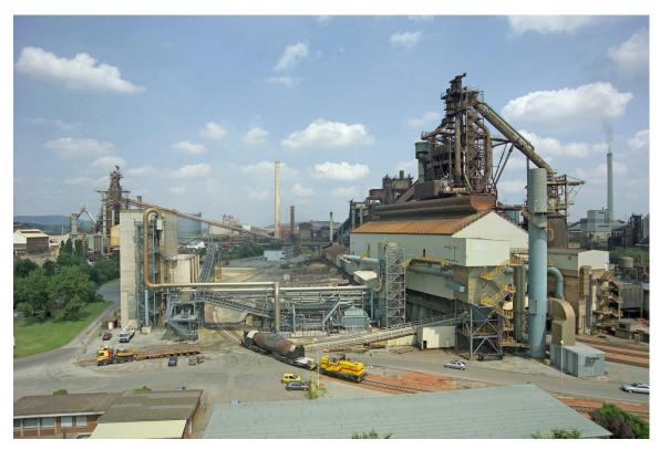
Blast furnace 4, of ROGESA Roheisengesellschaft Saar mbH in Dillingen, Germany. In conjunction with the relining of the blast furnace, Primetals Technologies will renew the electrical, measuring, analytical and automation equipment (Copyright: Dillinger Hütte).
