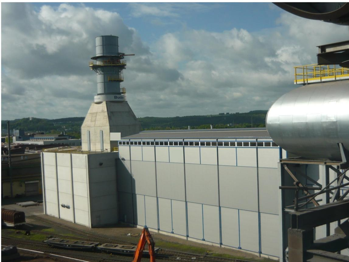
Outdoor dedusting facilities from Primetals Technologies on the Wetzlar site of Buderus Edelstahl GmbH in Germany. With a cleaning capacity of 2.4 million working cubic meters per hour, it is one of the largest systems of its kind in the world. It achieves a clean gas dust content of less than one milligram per standard cubic meter.
