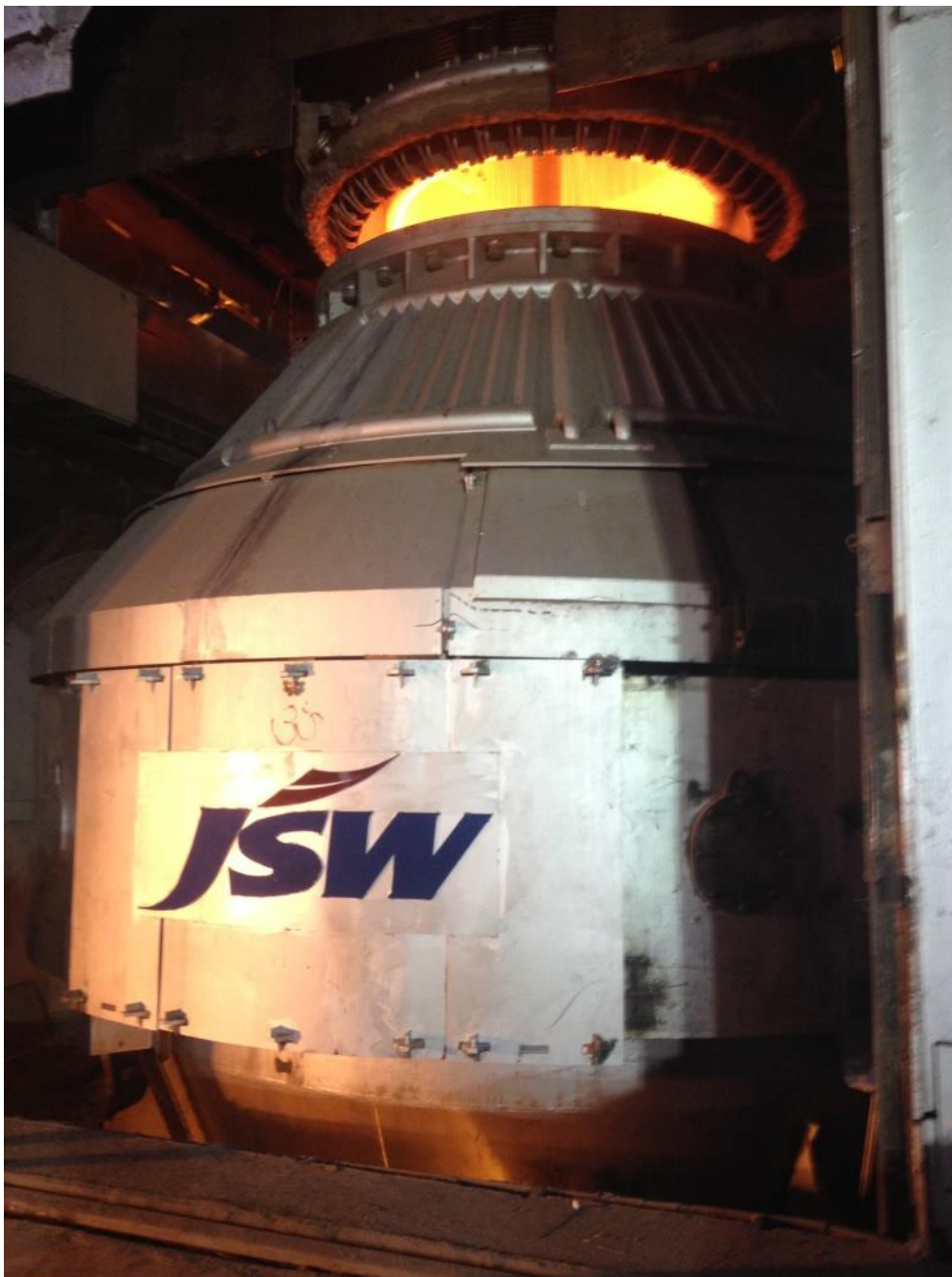
LD (BOF) converter from Primetals Technologies in the Steel Melt Shop no. 2 in Vijayanagar, Toranagallu, India of JSW Steel.
