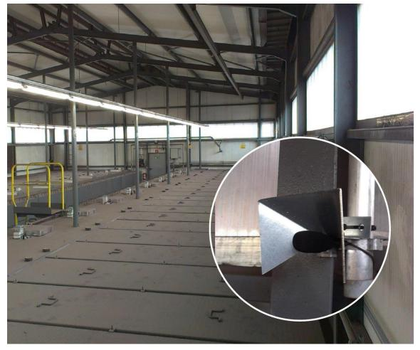
Bag filter housing and industrial microphone. Acoustic Expert measures and analyzes the sound spectrum to facilitate a condition-based maintenance strategy.
