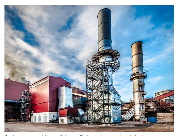
Outdoor systems of the new Primetals Technologies secondary dedusting system at voestalpine Stahl Gmbh in Linz, Austria. It achieves a clean gas dust content of less than one milligram per standard cubic meter (photo: voestalpine).
