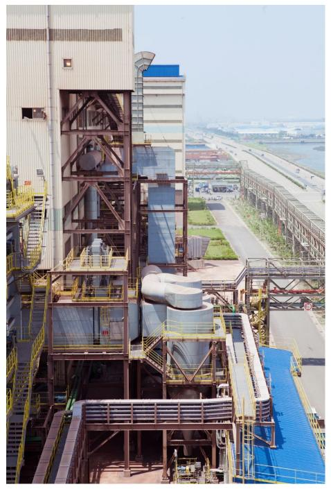
Selective waste gas recirculation (SWGR) system from Primetals Technologies
