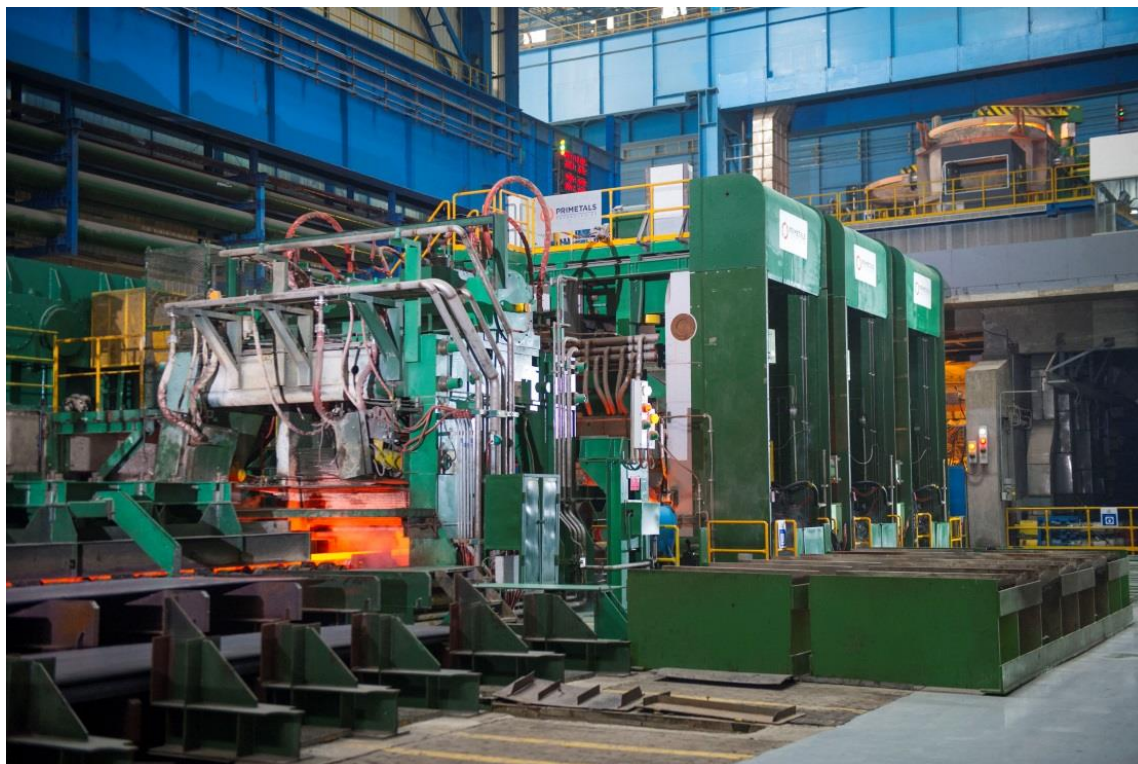
ESP Line Number 2 from Primetals Technologies in Operation at Rizhao Steel
