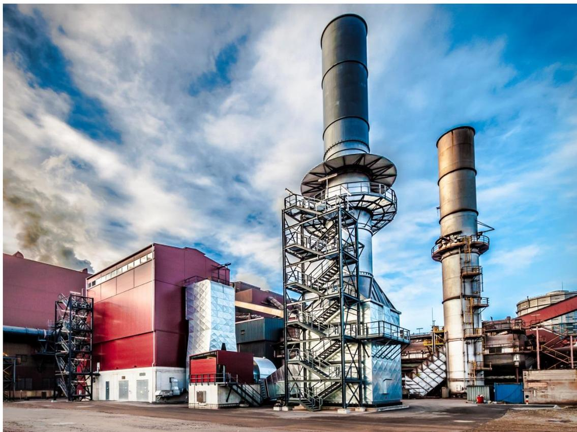
Outdoor systems of the new Primetals Technologies secondary dedusting system at voestalpine Stahl GmbH in Linz, Austria. It achieves a clean gas dust content of less than one milligram per standard cubic meter (photo: voestalpine).
