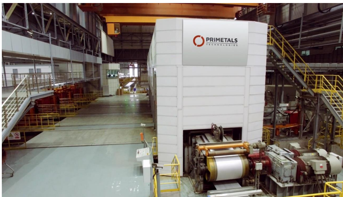
Cold rolling mill supplied by Primetals Technologies at Tangshan Iron and Steel Group Co. Ltd.
