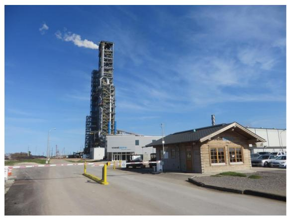
Midrex direct reduction HBI plant of voestalpine near the city of Corpus Christi, Texas on the Gulf of Mexico. The largest single module of this type worldwide was built by Primetals Technologies and Midrex Technologies, Inc. and achieved the performance guarantee test parameters in February 2017 (Photo courtesy of voestalpine).
