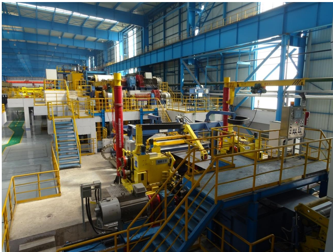
Side trimming section of the continuous pickling line from Primetals Technologies at Rizhao Steel Group Co., Ltd in Rizhao, Shandong Province, China
