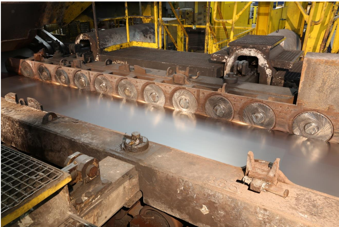
Side guides with Eco Slide Disc beams from Primetals Technologies at the entry side of the down coiler unit in the hot strip mill of voestalpine Stahl in Linz, Austria.
