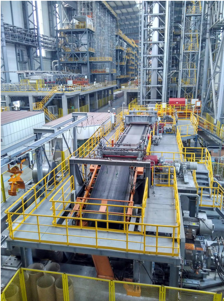
Continuous galvanizing line (CGL) from Primetals Technologies
