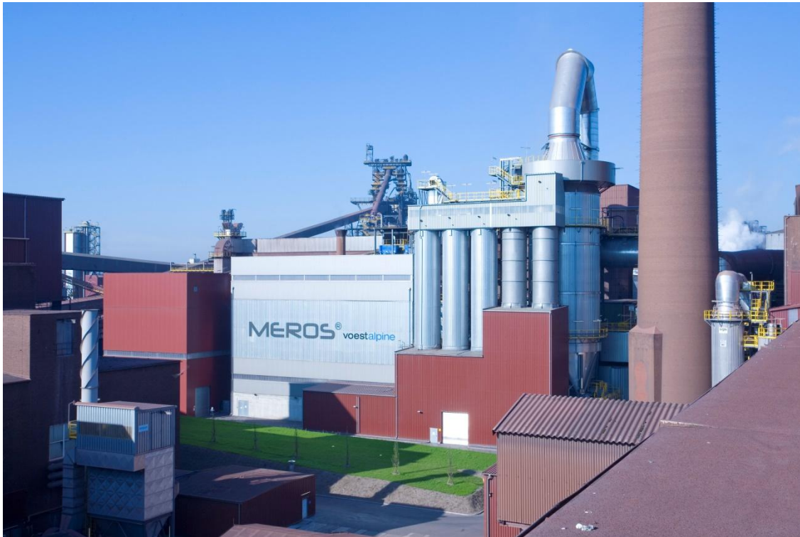
Meros plant from Primetals Technologies at voestalpine Stahl GmbH in Linz, Austria.
