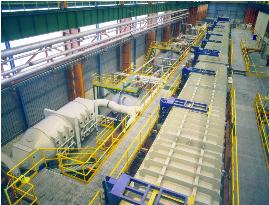
Continuous pickling line (CPL) from Primetals Technologies
