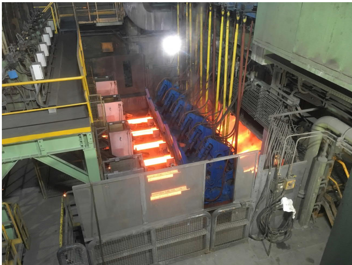
Continuous billet caster modernized by Primetals Technologies in the Lonato del Garda, Italy works of Feralpi Siderurgica
