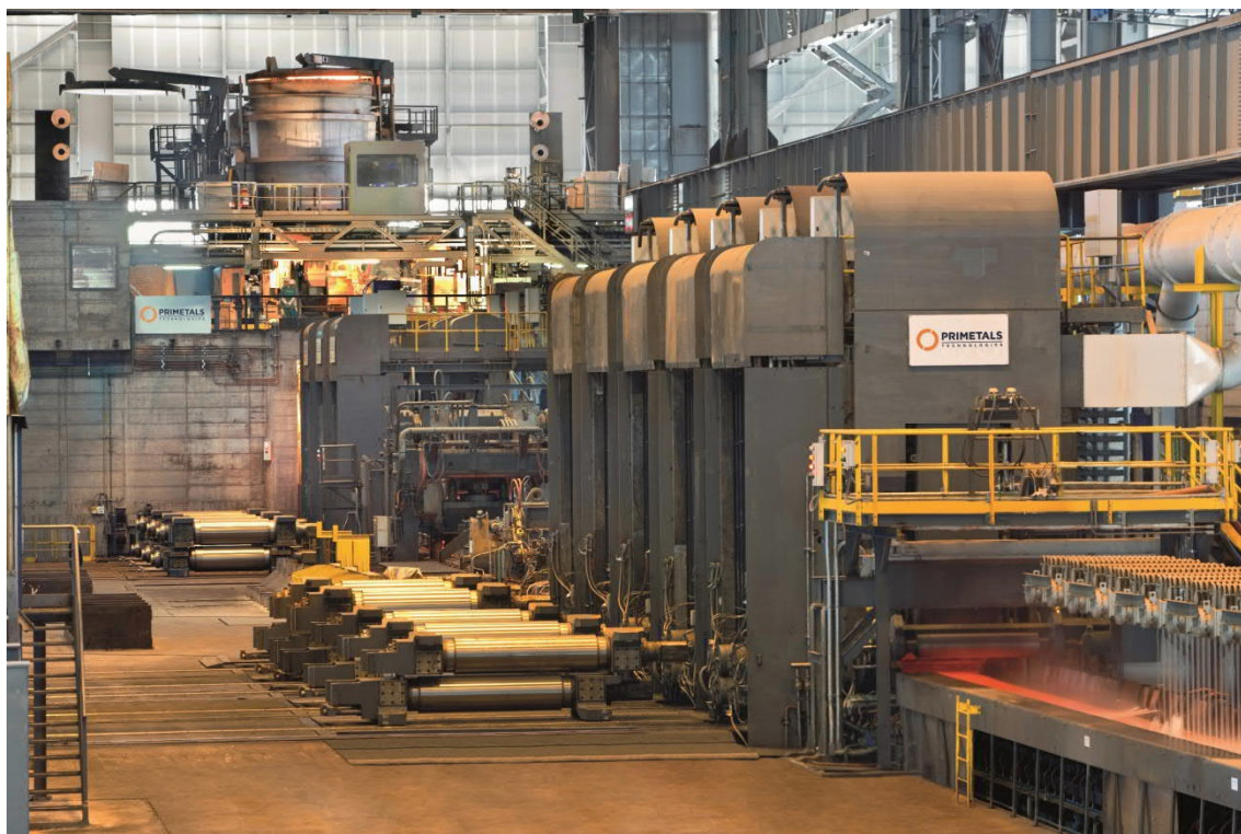
Arvedi ESP plant in operation
