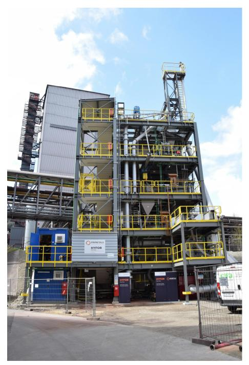
Photo of the HYFOR direct reduction pilot plant for iron ore fines developed by Primetals Technologies and located at the voestalpine site in Donawitz, Austria. The DR process is CO<sub>2</sub>-free and H<sub>2</sub>-based.
