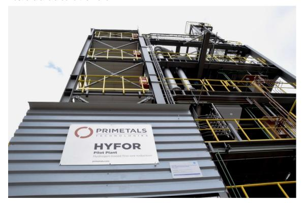
Photo of the HYFOR direct reduction pilot plant for iron ore fines developed by Primetals Technologies and located at the voestalpine site in Donawitz, Austria. By joining the Heavy Industry Low-Carbon Transition Cooperative Research Centre, MHI Australia and Primetals Technologies will help Australia's iron and steel sector to decarbonize.
