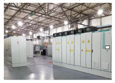
Primetals Technologies has upgraded the Nucor Hickman hot strip mill F5 and F6 main drives, pictured here in the foreground.
