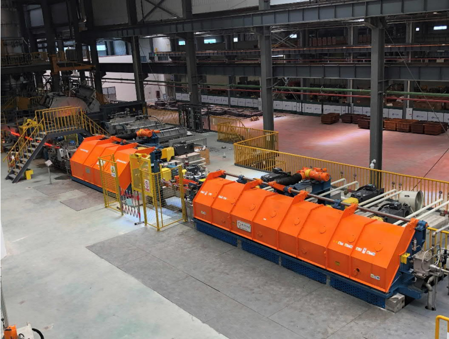
Copper rod mill from Primetals Technologies.
