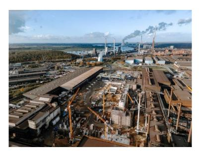
With the laying of the cornerstone for the construction of a modern hot-strip mill, the conversion and construction of two continuous casting plants, and the construction of two new walking beam furnaces, thyssenkrupp Steel is taking decisive steps to strengthen its position in European competition. Photo copyright: thyssenkrupp Steel.
