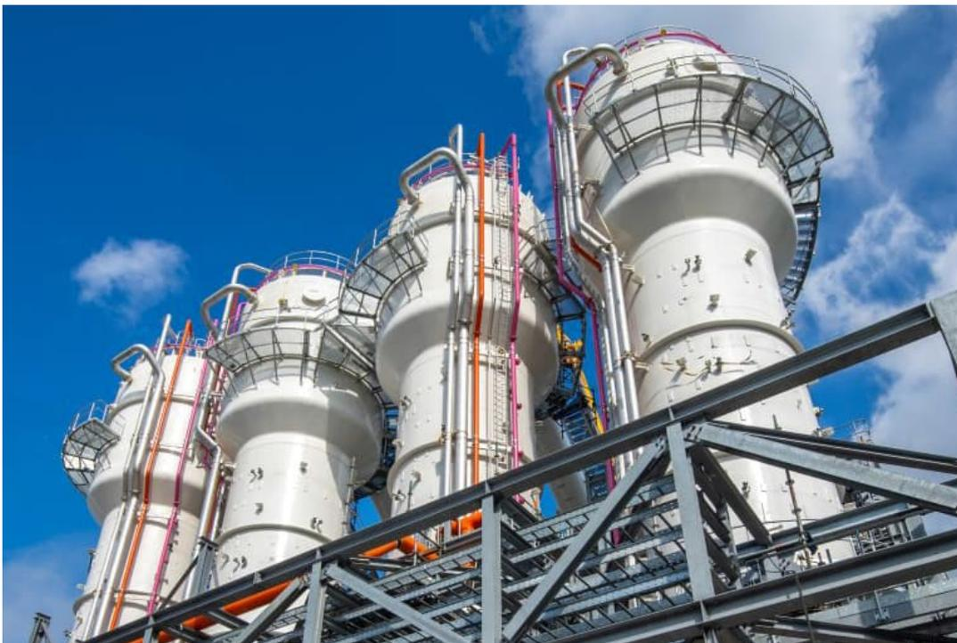
A key part of the Steelanol plant, the bioreactors is where ethanol is produced.
