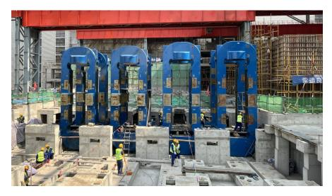
All four high-reduction mill stands were installed on site as part of a record-setting project execution timeline.
